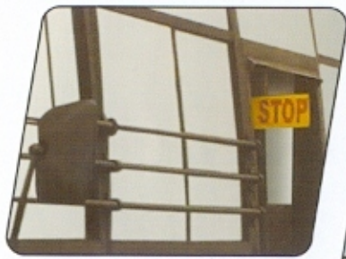
Window railings for safety
